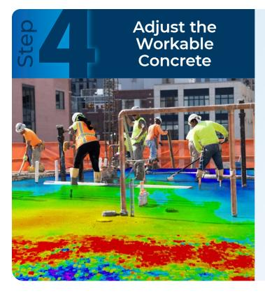
Thanks to the Flatness Check<sup>™</sup> App, operators can easily identify – with pinpoint accuracy – any swells and dips in the concrete slab. Armed with this data, the team can perform the following tasks:
